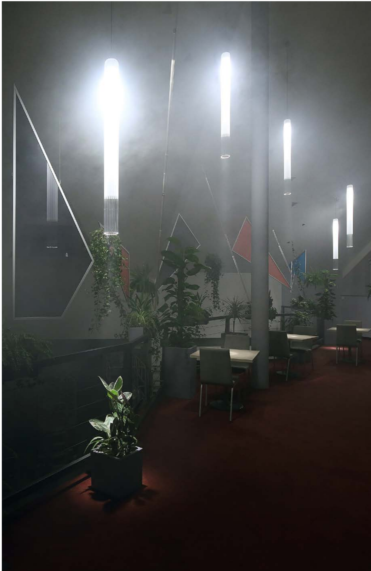
PRIVATE COMPANY TUBES INSTALLATION
